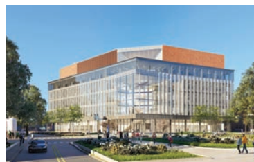
Groundbreaking, November 2022, Stanley R. Zupnik Hall Interdisciplinary engineering building University of Maryland, College Park
