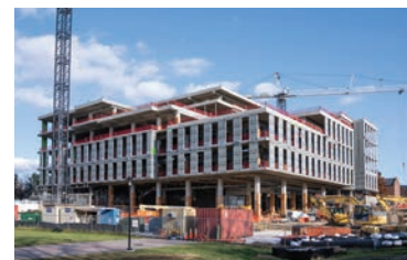
Under Construction, 2022 College of Health Professions Building Towson University
