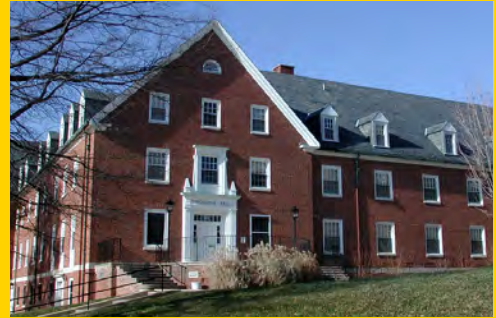
Dorchester Hall Renovation (2018)
